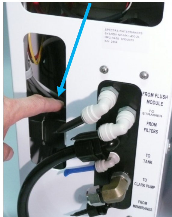
Push Diversion valve button down and turn 90 degrees to manually open valve.
