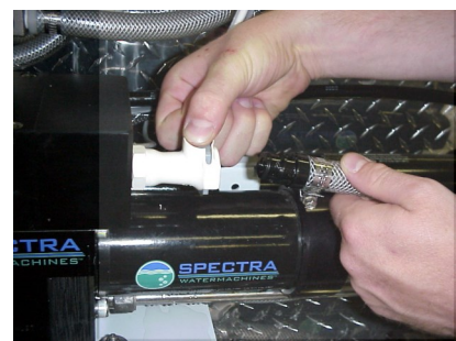
Connecting brine discharge service hose
