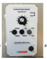
The VFD (Variable frequency Drive) speed control for the optional boost pump can be mounted on a wall near the Watermaker control box or can be mounted to the frame of the unit.
