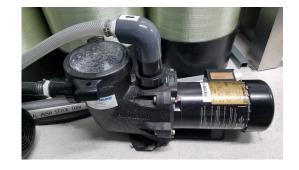
microns and supplied at 19-21 GPM and regulated between 10-25psi. The actual boost pressure requirement will be determined when commissioning the system and should be set as high as possible without causing the Pearson Pump to knock. The final boost pressure setting depends on the final installation configuration.
